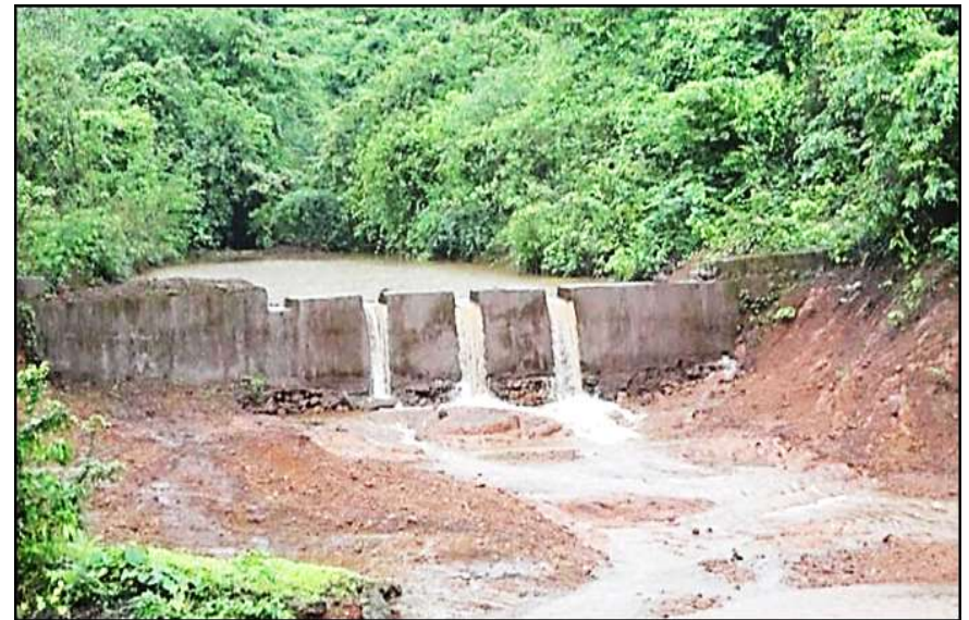
Environment Management: Provision of Filter Beds & RCC Silt Arresters
