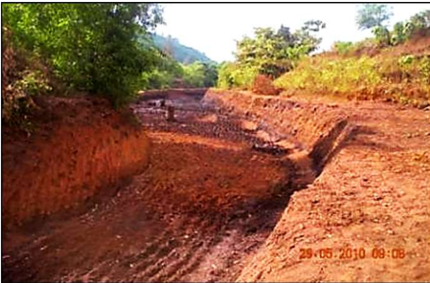
Monsoon Preparations: De-silting of Garland Drains & Settling Ponds
