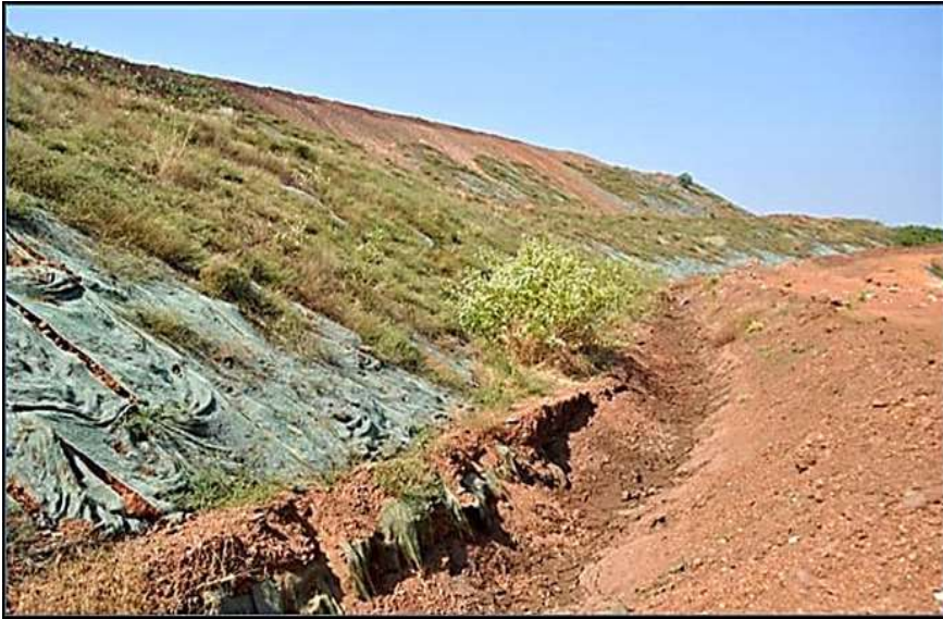
Environment Management: Provision of Garland Drains at the Dump Toe
