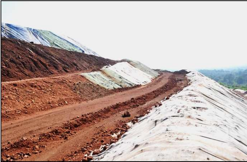
Erosion Control: Contour Drains for Water Channelization
