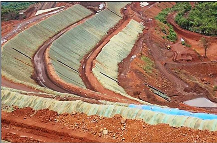
Laying of Geotextile for Erosion Control
