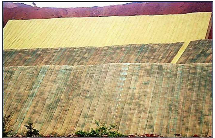
Laying of Geotextile for Erosion Control
