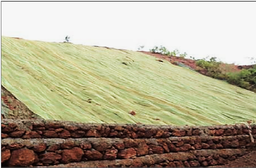
Protection Measures: Provision of Boulder / RCC Wall
