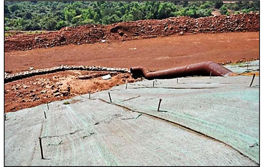
Erosion Control: Provision of ERWMS Pipes
